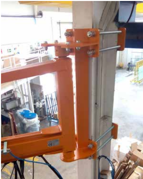
METAL COLUMN WELDING + REINFORCED BRACKETS
